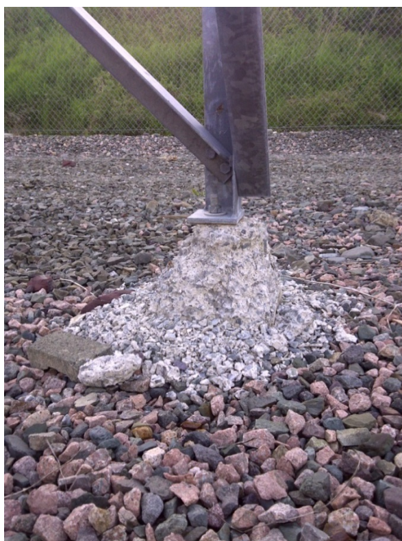
Figure 13: Structure L01L37-1 Western Avalon Terminal Station
