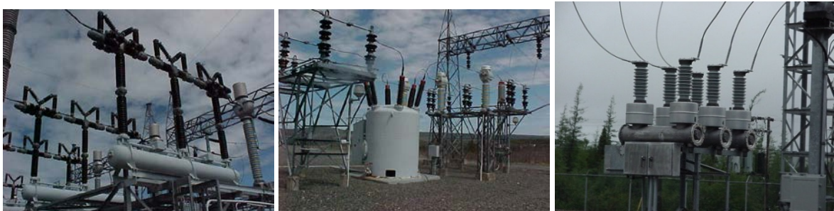
Figure 9: Circuit Breakers – ABCB (left), Oil (middle), and SF 6 (right)
