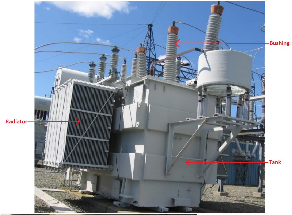
Figure 8: Power Transformer
